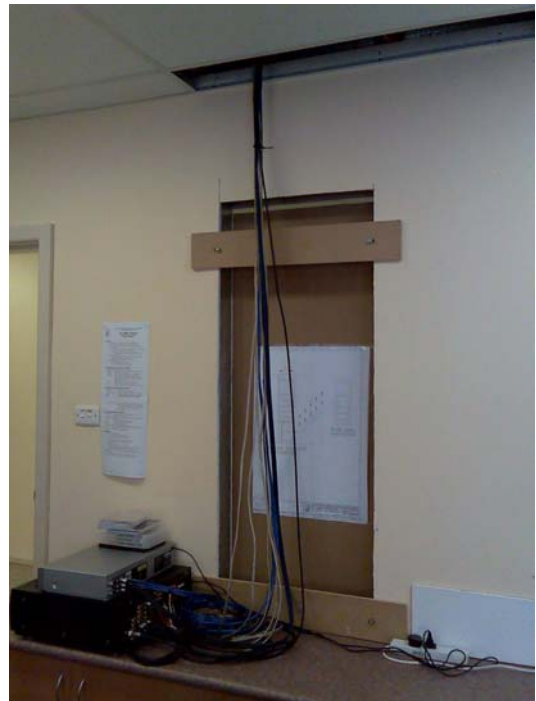
The cutout has been created in the office wall for the permanent installation of the Audio / Visual equipment. A cabinet accessible from both sides of the wall will be installed in this hole.
